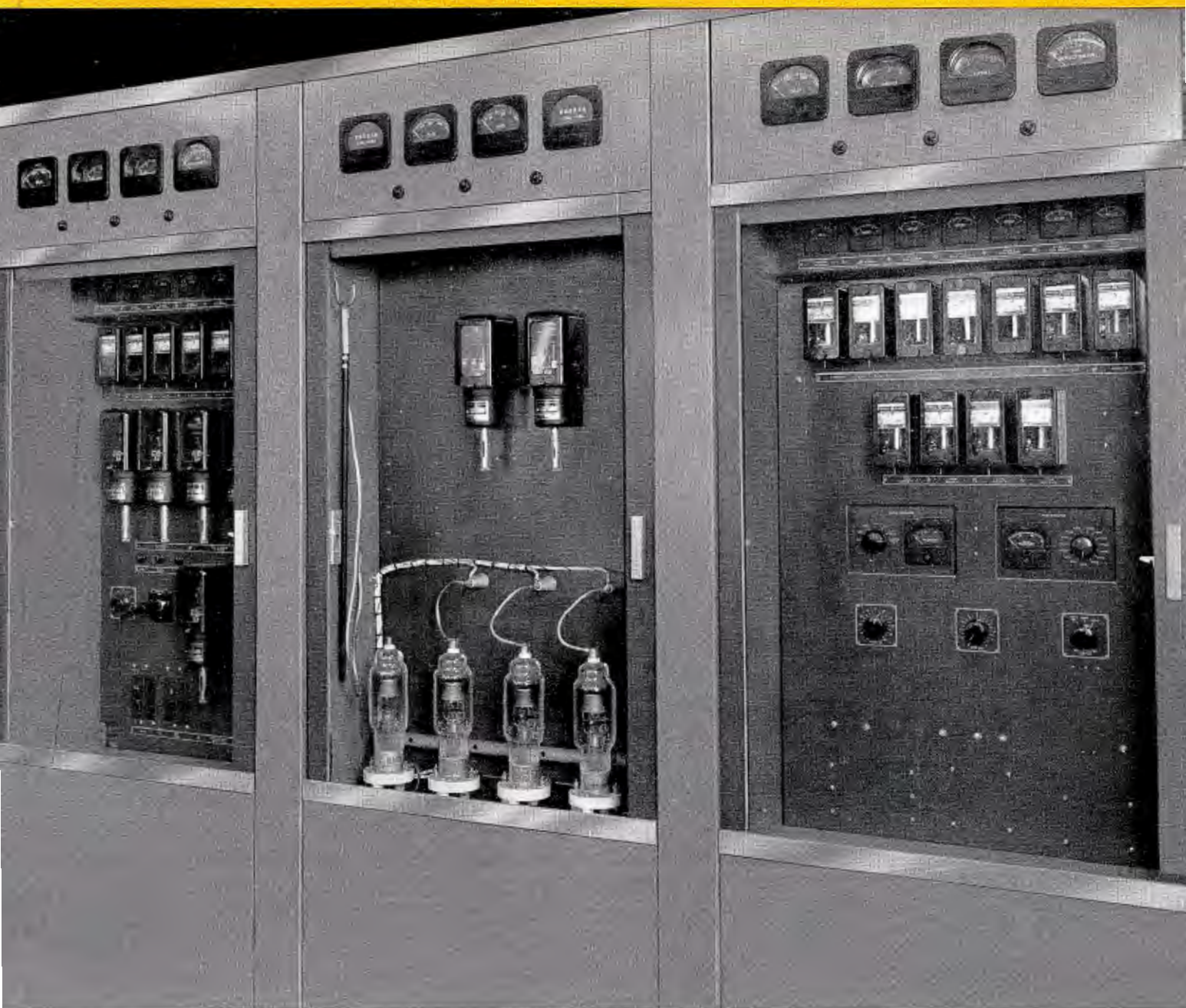
Central cabinets of the 10 kw driver showing control and distribution, screen rectifier, and regulator units.
