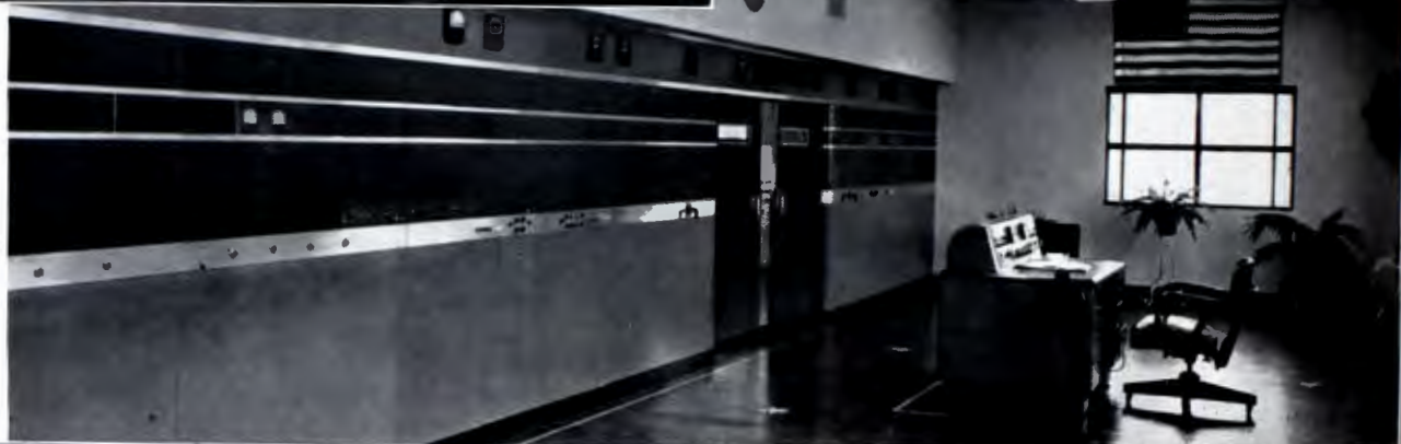
Fifty kilowatt transmitter, Type BTA-50F, with control console and extension cabinets containing phasing equipment, at KMPC, Hollywood, Cal.
