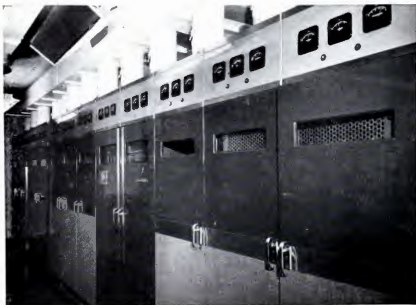
WENR-TV. The RCA 5-kw television transmitter Type TT-5A and RCA 10-kw FM transmitter Type BTF-10B at WENR-TV. This station also includes an RCA Superturnstile antenna, field truck and field camera equipment, studio cameras, video and audio control-room equipment, film projectors, film cameras, turntables, and microphones.
