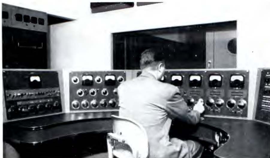
KOMO, Seattle. This master control console—with 9 deluxe audio equipment racks (at rear, not visible)—is one unit of KOMO's completely new and modern 7-studio system. It incorporates complete center panel switching for 10 studios and 6 outgoing channels (KOMO-AM, KOMO-FM, network plus 3 emergency).
