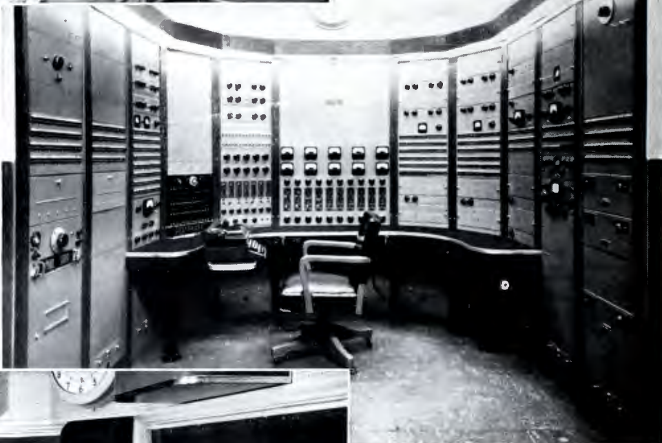
WNEW, New York. This master control installation in WNEW's 7-studio lineup is flanked on each side by 5 deluxe audio equipment racks. It has complete facilities for control and preset switching of 7 studios to 10 outgoing lines . . . and for feeding cue from any channel to any studio.
